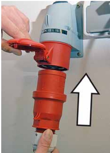
Fig.23: Connecting welder to power supply
